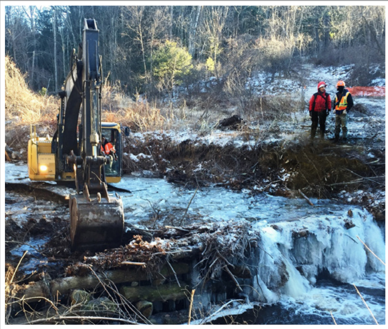
Timber Dam removal, Amethyst Brook, Pelham
